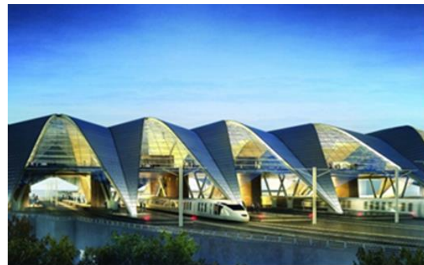
10.2.att. Rail Baltica
