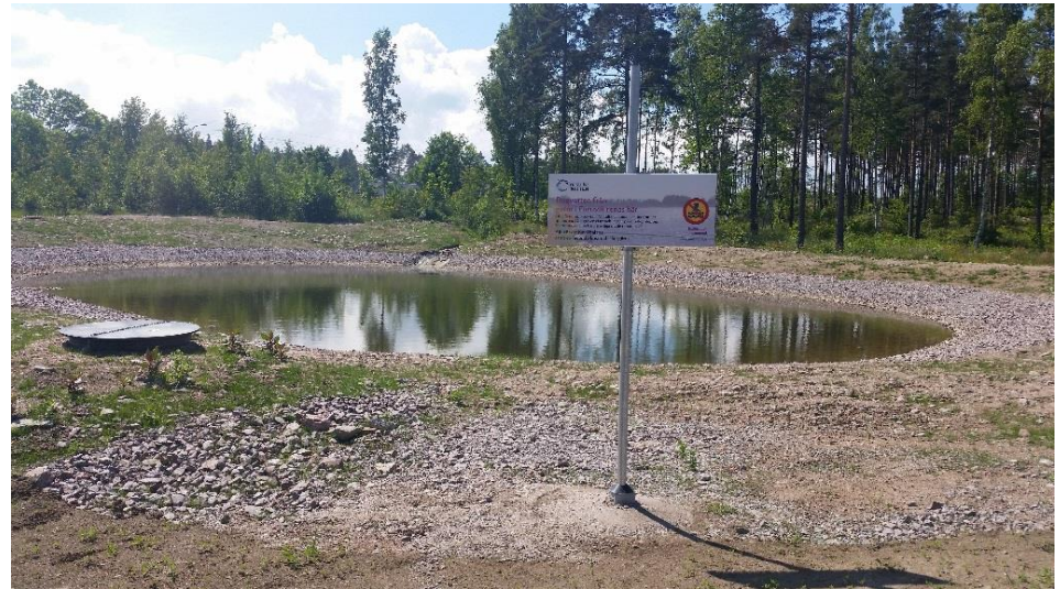
Storm water pond– outside Gävle City Main target: Retention and cleaning of storm water before outlet in sea
