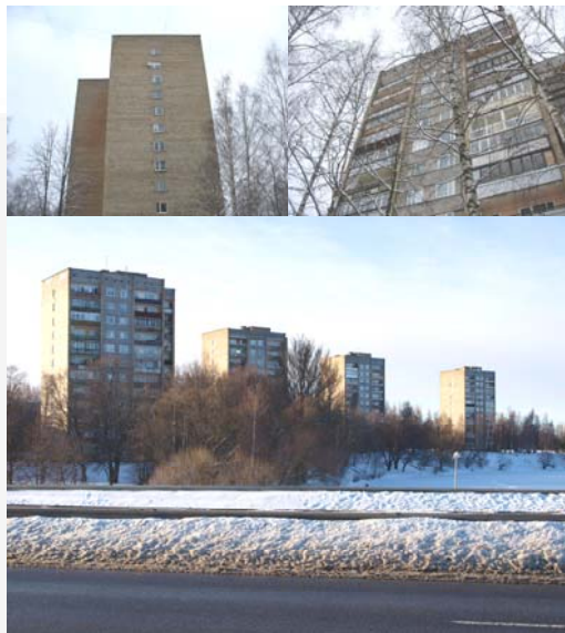
Pic.17, 12-floor multi-apartment buildings in Jugla
