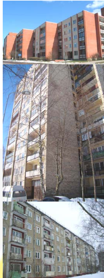
Pic.6, typical multi-apartment buildings in Jugla
