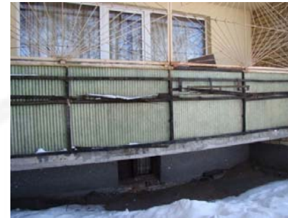
Pic.12, Loggia of a 12-floor multi-apartment building in Jugla [2]
