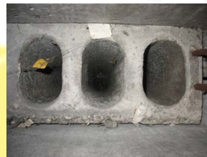
Pic.14, clean ventilation shafts (multi-apartment building of series No.464). [7]
